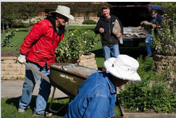
The Work Crew installs pavers for the garden patio.
